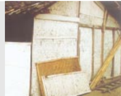
Plastered walls in Costa Rica
