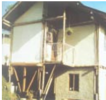
Plastered walls in Costa Rica
